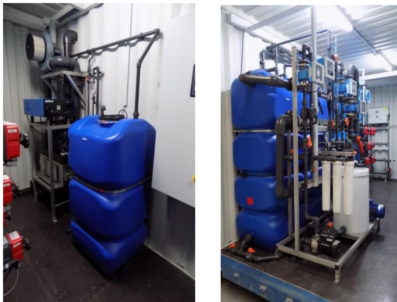
Figure 12. Container assembly photos
