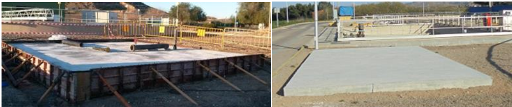
Figure 17 Concrete slab works. Figure 18. Concrete Slab finished
