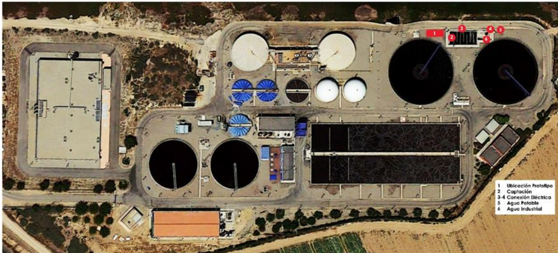
Figure 16. Location of the pilot plant in Cabezo Beaza WWTTP.
